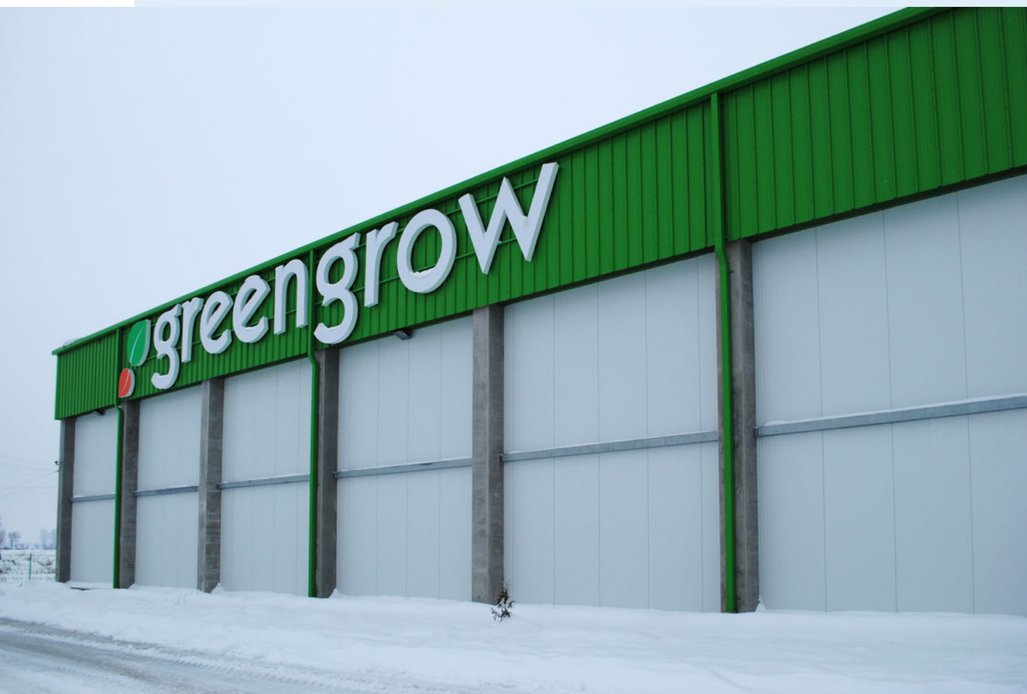
The new Greengrow storage hall in Wikrowo, Gronowo Elblaskie
